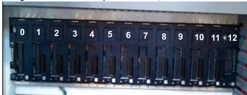
Figure 9: The New Backplane Installed, With Slots Numbered
